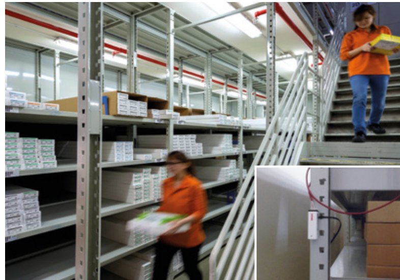
RMS Mini Logger installed in the warehouse.
